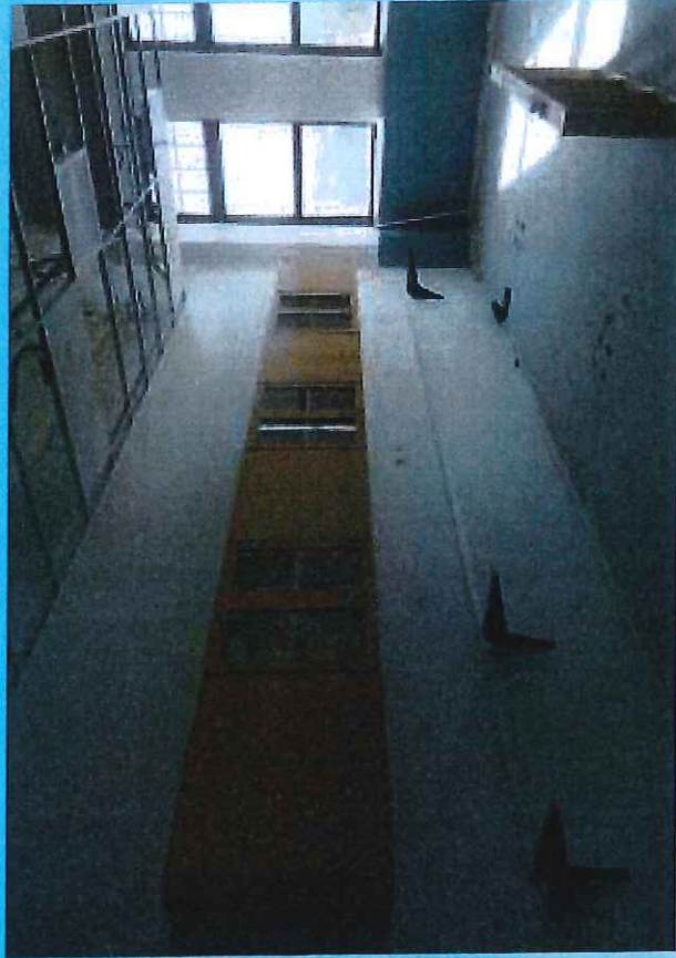
West Wing 2 nd Floor Cabinet Installation
